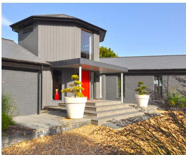
FRONT The brick bungalow has been rendered, with a new roof and aluminium-framed windows. The entrance was redesigned to create a canopy above a new red front door leading into the tower.
