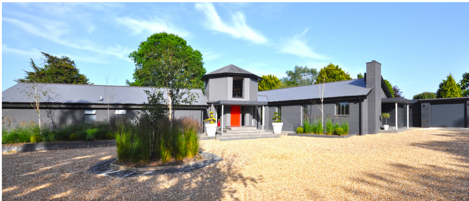
FRONT The brick bungalow has been rendered, with a new roof and aluminium-framed windows. The entrance was redesigned to create a canopy above a new red front door leading into the tower.
